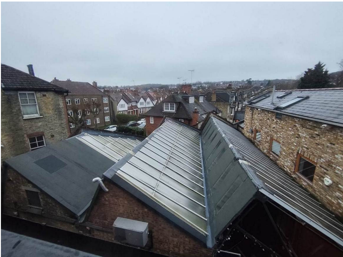
Figure 6: Roof over courtyard minimises noise breakout to surrounding area. NB: live/work units are on the right and the upper floor windows are shielded by the roof structure over the courtyard
